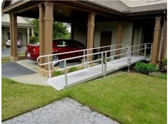
Ramp modification through King County Home Repair Program
