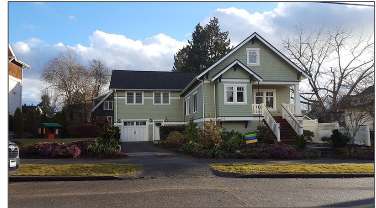
Seattle garage conversion to attached ADU. (Photo Credit: Sightline Institute)
