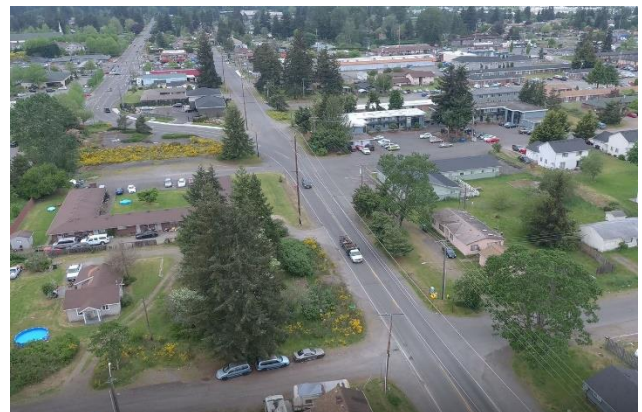
111 th and 112 th Street Corridors
