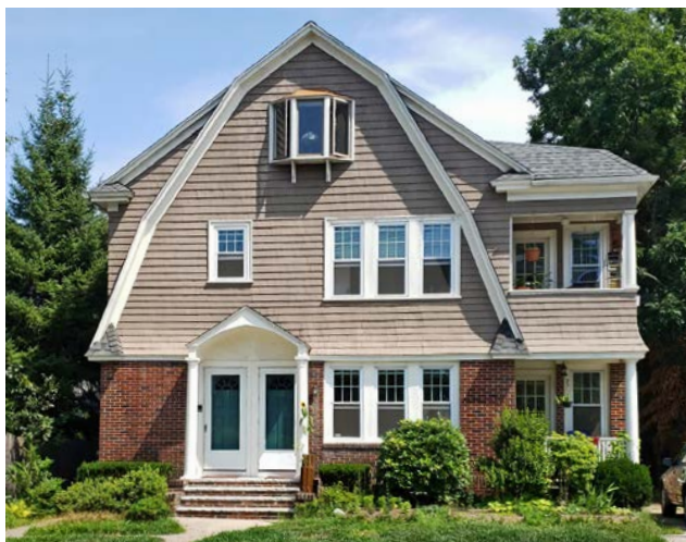
▲ Providence, Rhode Island, has many homes that were built as or long-ago converted into multidwelling units. (Notice the two front doors.) A homeowner can live in one apartment while renting out the other.
