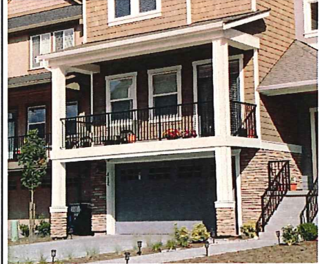
A balcony over garage with decorative support columns.
