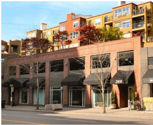
Figure E.8.1.b. This building uses openings on its second level parking area to resemble windows.
