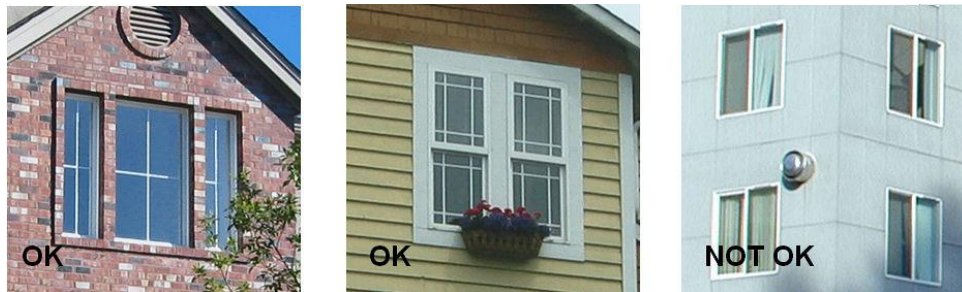
Figure E.5.1.b. Examples of window details. The two on the left employ trim, multiple panes and window groupings. The one on the right provides no refinement or sense of quality.
