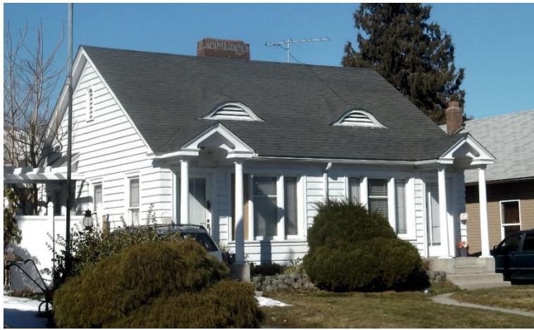
Figure E.3.1.a. This attractive duplex is in one of Wenatchee’s predominantly single family neighborhoods and articulates a simple rectangular floor plan with porches, window patterns, and eyebrow windows.
