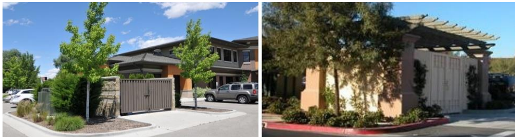
Figure C.7.2.a. Both examples use durable and attractive enclosures with trees and shrubs to soften views of the enclosures from the side. The right example uses a trellis structure on top – a desirable example particularly where the top of the enclosures are visible from surrounding buildings, streets, and pathways (due to topography or building heights).
