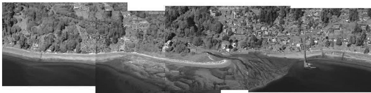
Figure 1 – Series of four photos illustrating continuity of coverage and typical overlap between images.
