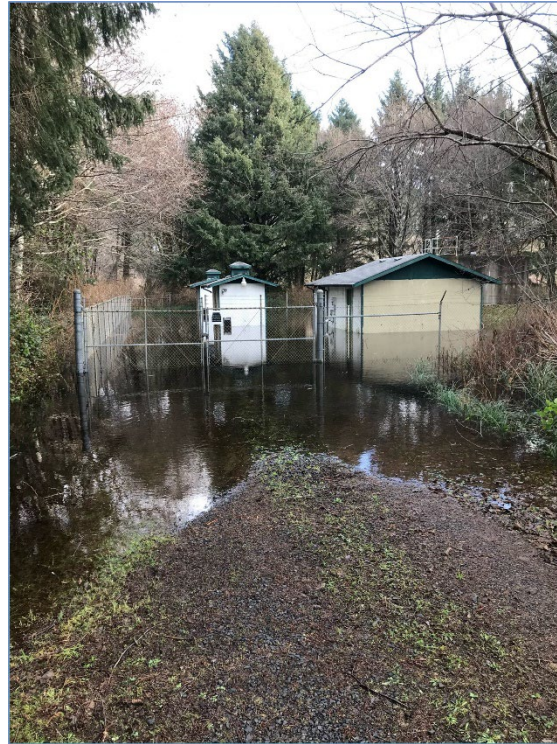
Grays Harbor County Utilities Department Water Well, 1-07-2022
