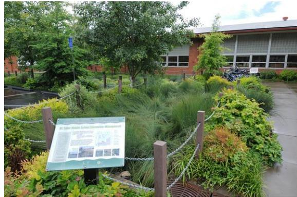
**Purpose:** These projects would reduce stormwater runoff from a large, impervious area. This would reduce stormwater runoff volumes and decrease peak flows that are currently conveyed through the stormwater drainage system.
