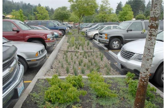
**Purpose:** This project would reduce stormwater runoff from a large, impervious area that eventually discharges to Alder Creek. This would reduce stormwater runoff volumes, decrease peak flows, and reduce pollutant loadings that are currently conveyed through the stormwater drainage system to the creek.
