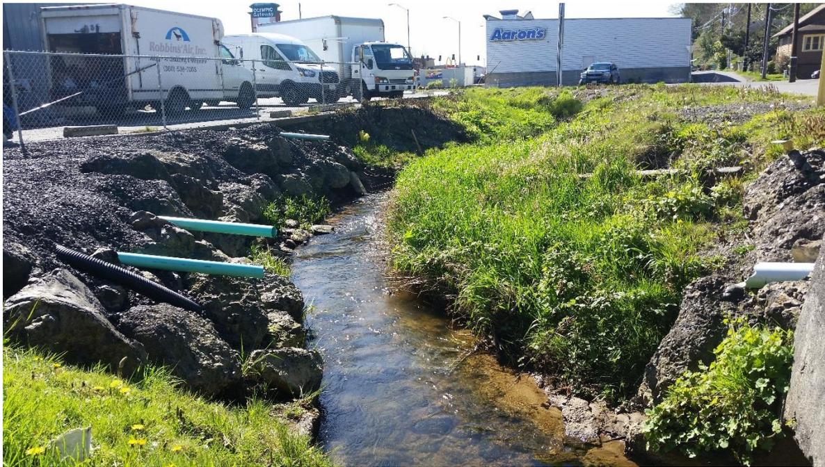
**Flood Benefit:** Local residents and City of Aberdeen Public Works staff have stated that flooding often occurs in the lower reach of Wilson Creek. Removing or replacing culverts with larger crossings would address assumed flow restrictions on Wilson Creek, reducing upstream flooding frequency and depth.
